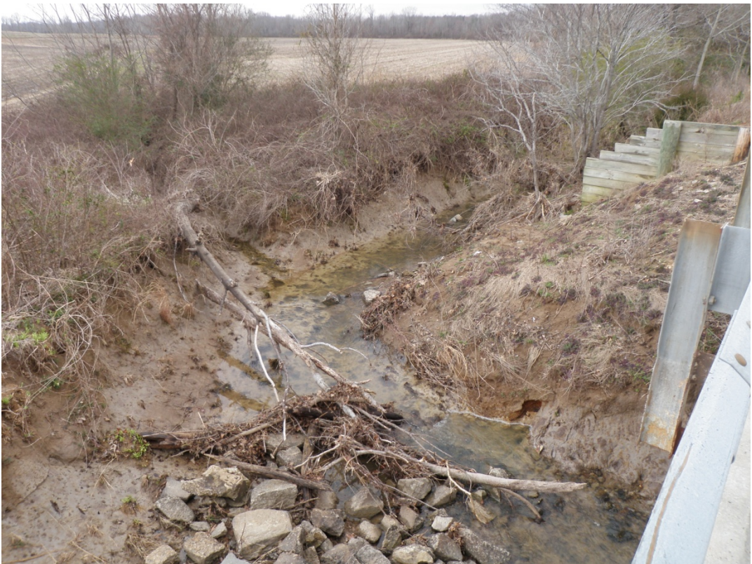
STR-1 Looking Upstream
