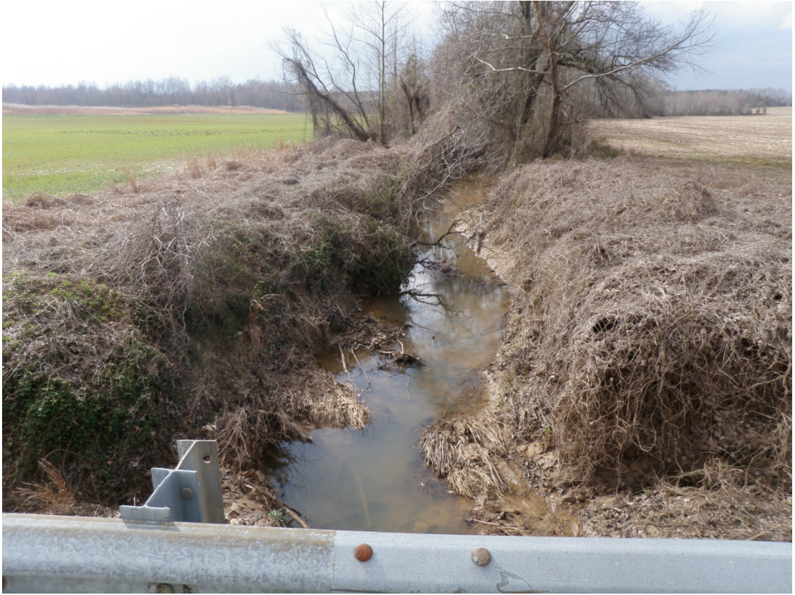
STR-2 Looking Upstream
